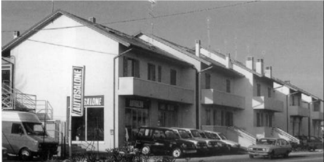
Picture 1 – Building units erected by the Emmedue building system
