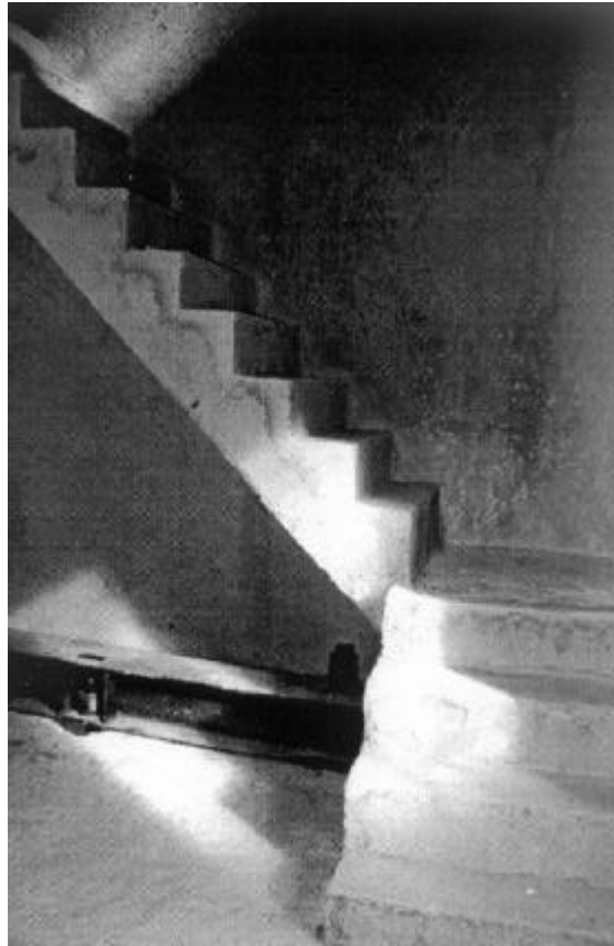
Picture 8 – The staircase inside the prototype
