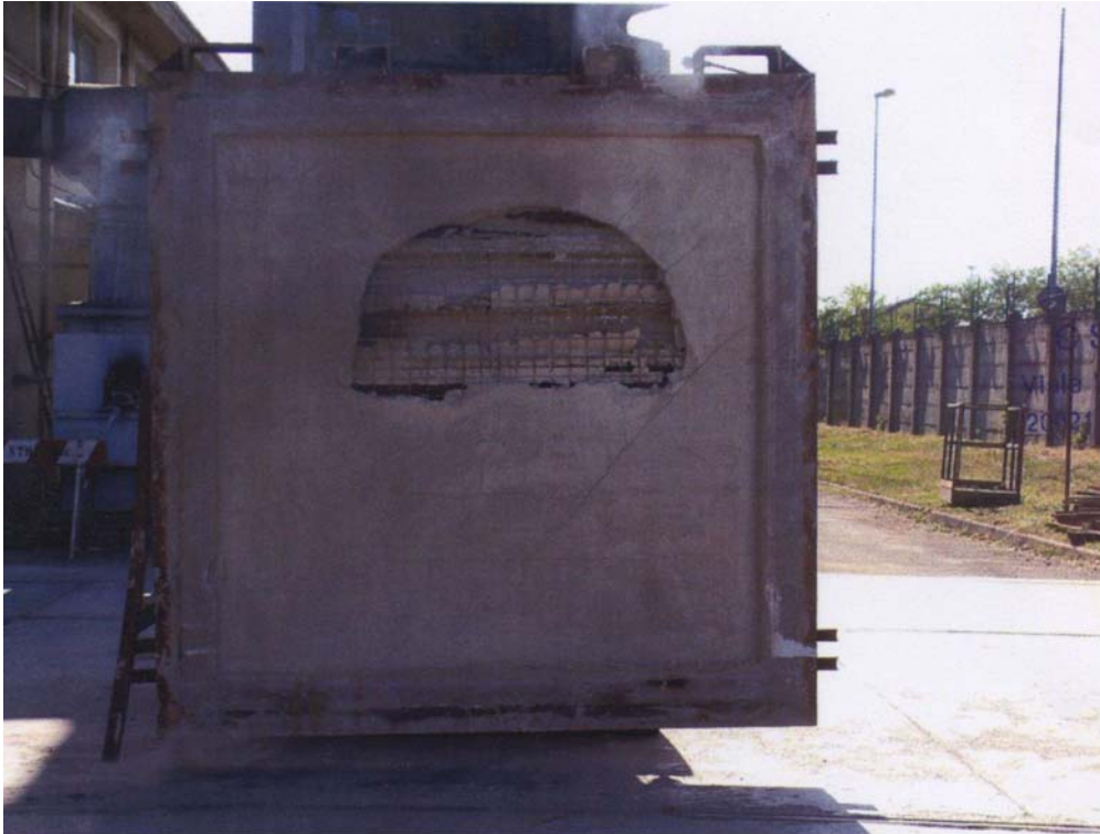
Photo 3: element side exposed to fire after testing
